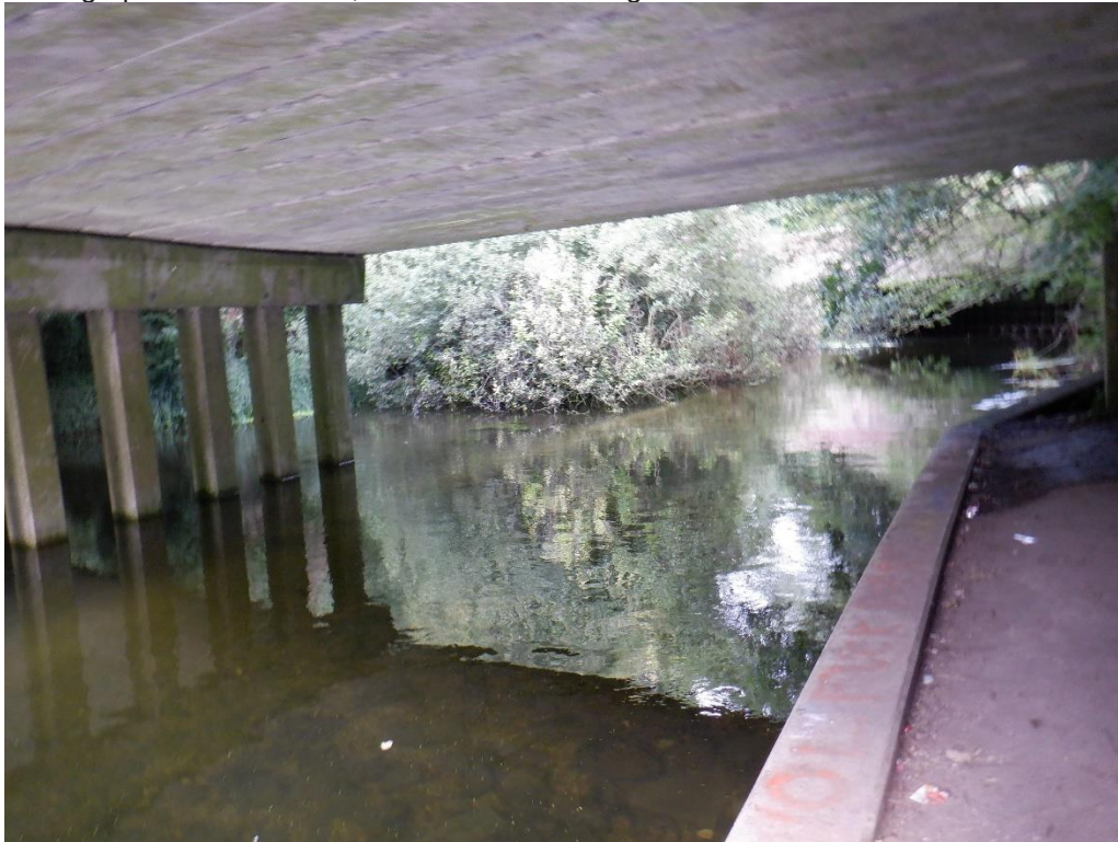
Photograph 3. River Itchen, under A34 road bridge
